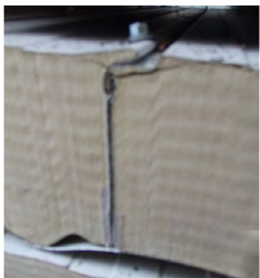
Figure 3: Panel-to-panel joint of JI PERMAPAN 120 PIR
