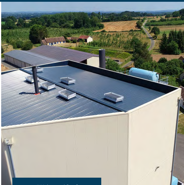
Jl Vulcasteel Roof
